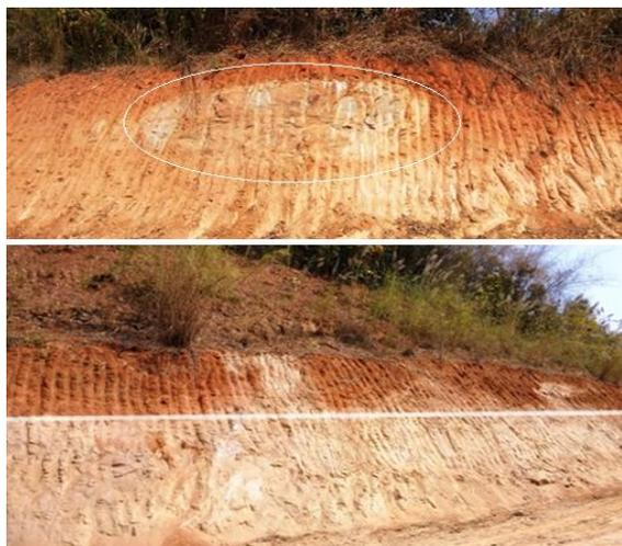
Figure 1: IITG Cut Slope Site depicting two layers of soil and weathered corestones. (Top layer is referred as SOIL 1 while the bottom layer as SOIL 2
