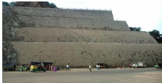
**Fig.1** Four tier MSE wall of 44 m height
