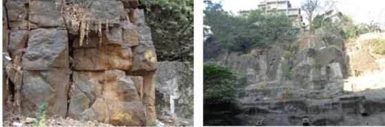
Fig. 1 The present Rock slope appearance on out crops from eastern to western corner of the slope (a) dominant joint sets, discoloration and staining of rock material due to weathering clearly visible (b) already stabilized portion of the rock slope.
